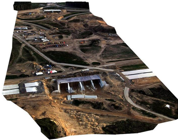
Figure 3: Digital Surface Model of Motorway interchange construction site [62].
